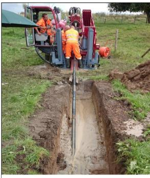
Installing the fiber cables by means of horizontal directional drilling
